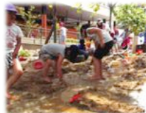
Using a well pump and watercourse together
